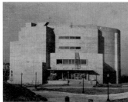
Recent Photograph of Aviation Medical Acceleration Laboratory showing construction work near completion.
