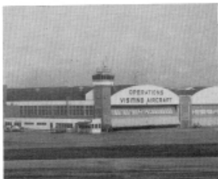
View of NADC Hangars from Airfield
