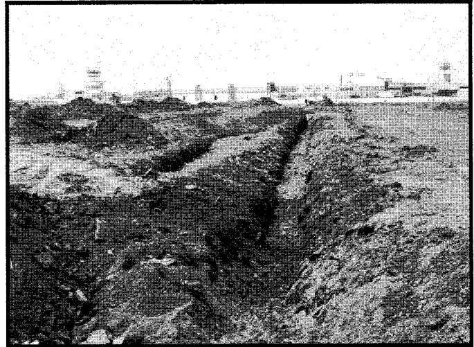
Trench for piping of groundwater to pump and treat facility.
