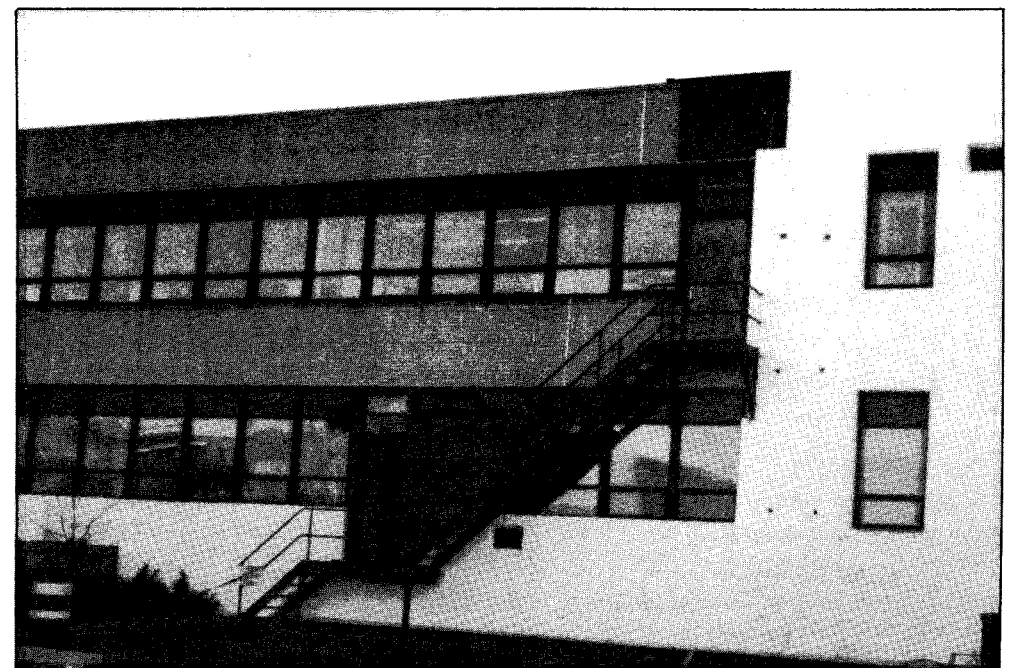
Building 3 receives renovation as part of total program.
