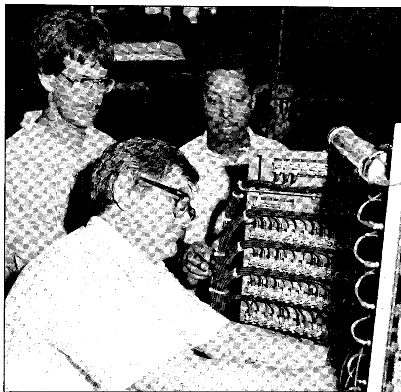
WIRED IN — Tom Haug and Jerry Duley watch Phil Huber put their electrical design into practice as he wires the P-3's control panel.
