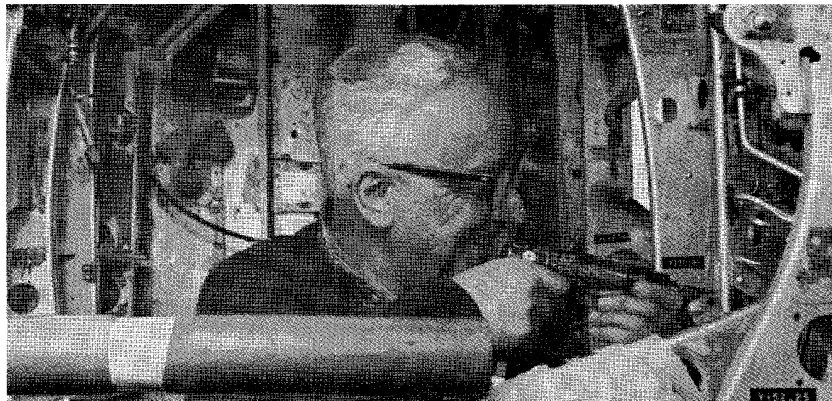
Craftsman Nic Tursi works on an RF-18A prototype aircraft installation.
