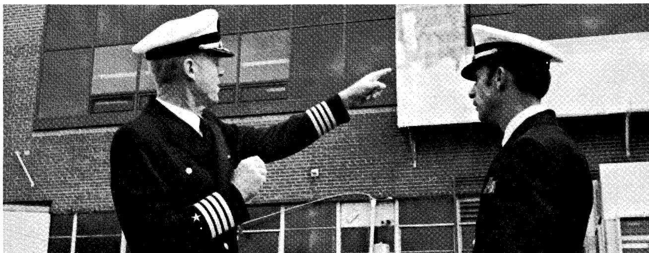
Public Works Officer LCDR Ray Tyler, rt, shows Center Commander, Captain James Anderson new windows that are part of NADC's energy conservation program.
